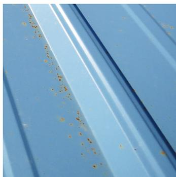
Example of red rust on the surface of a painted metal panel, caused by metal filings
